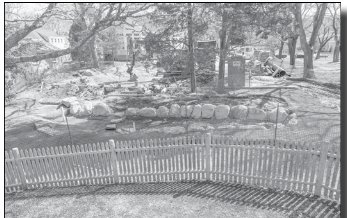
Installation of LSTA grant-funded stormwater bioretention garden
